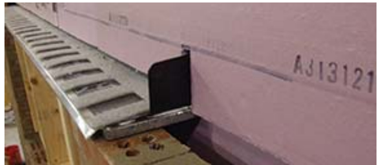
TotalFlash ® flashing preassembled unitized through wall flashing/drip edge assembly installed over continuous steel brick ledge.
