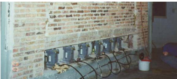
ASTM E119 Test Assembly, Exterior Side
